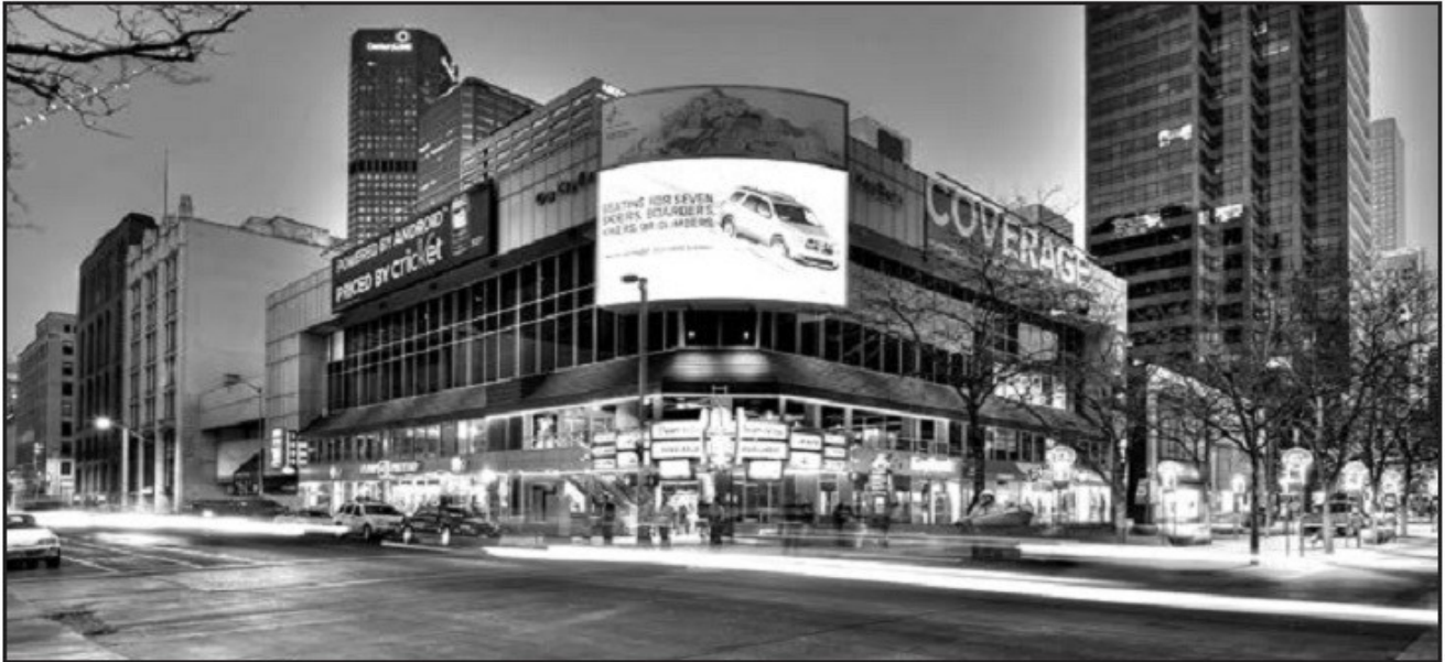
Champa Square underwent nearly $8 million in renovations in 2010.
